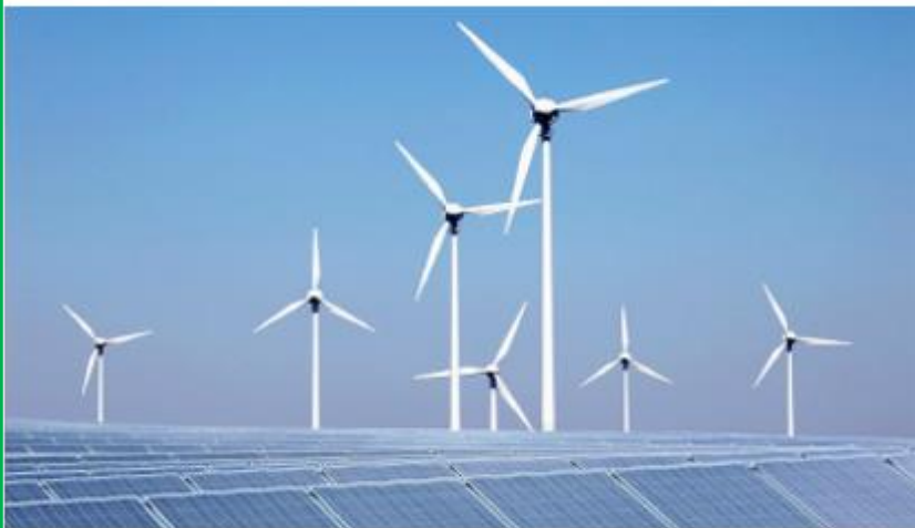
wind power generation
